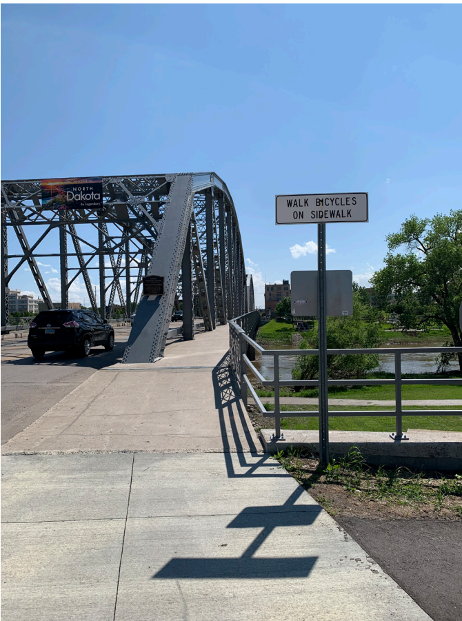
The Red River is a barrier to multimodal access between Grand Forks and East Grand Forks.
