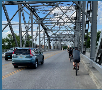
Bridges – The bridges that link Grand Forks and East Grand Forks are a challenge for cyclists.
